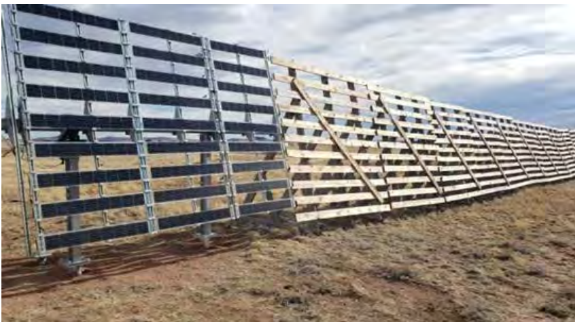
Snow fences with mounted solar in Minnesota.
