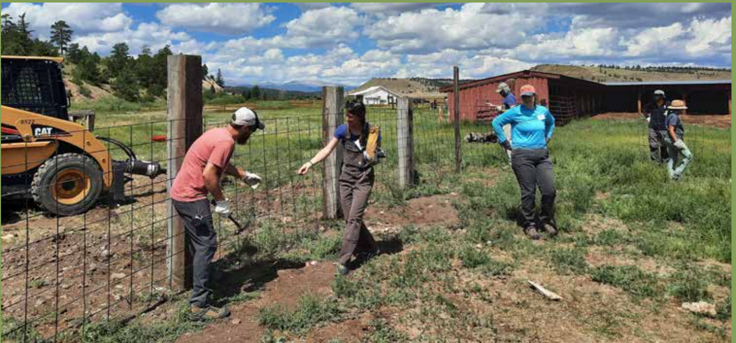
Volunteer day repairing fences at Santa Maria Ranch in Hartsel
